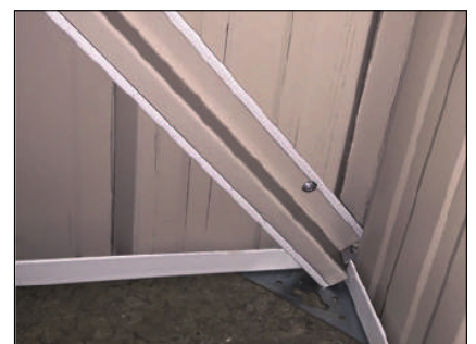
Wall Bracing - Bottom
