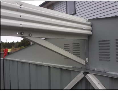
Ridge Beam connection to Gable
