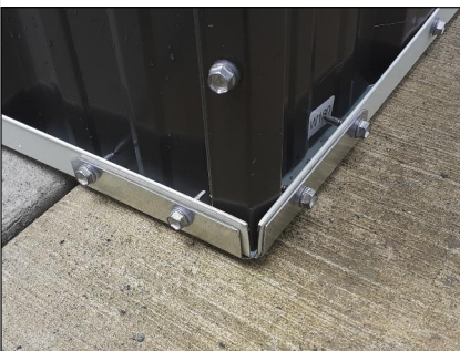
Corner Anchor Exterior - Bottom
