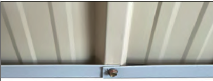
Ridge Beam connection to Gable
