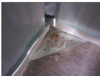
Corner Anchor Interior - Bottom
